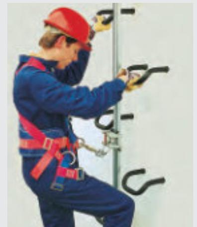
Fastening the fall arrest rails between the step irons
