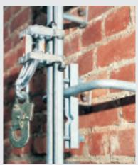
Fasteningthe fall arrest rails in the middle of the step irons
