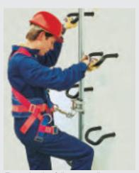
Fasteningthe fall arrest rails between the step irons
